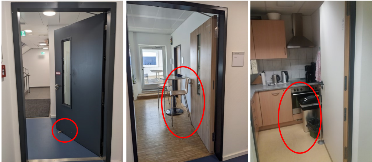
Figure 5: Decommissioning of a fire door
