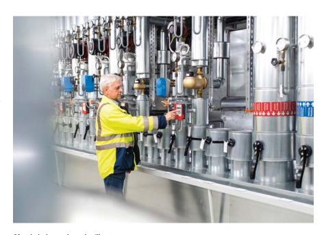
50 technical control panels will not only be completely refurbished but also optimally adjusted individually.
